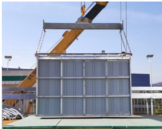
Figure 4 Lifting Membrane case
